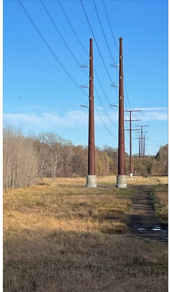
Two-pole structures for angles and dead-ends
